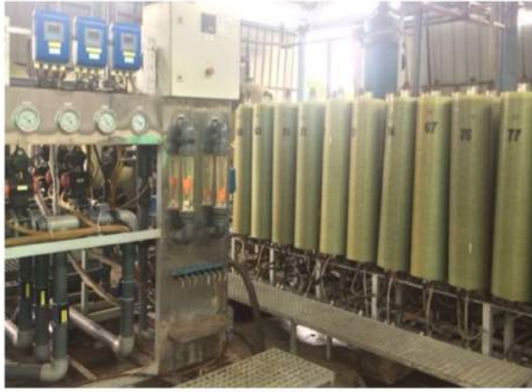
Reverse Osmosis Plant
