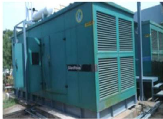
Acoustic Enclosures of DG Set
