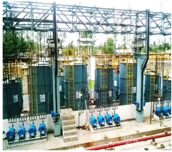
Primary And Secondary Condensers for VOC control
