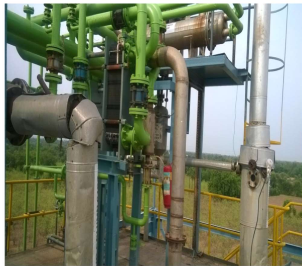
Primary And Secondary Condensers for VOC control
