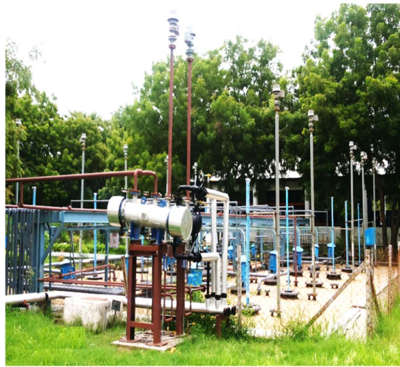
Primary And Secondary Condensers for VOC control
