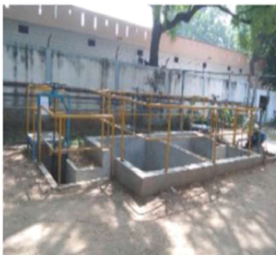
Guard Pond for Storm Drain
