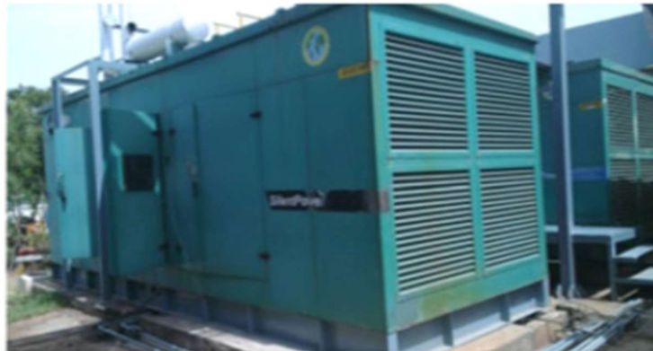
Acoustic Enclosures of DG Set
