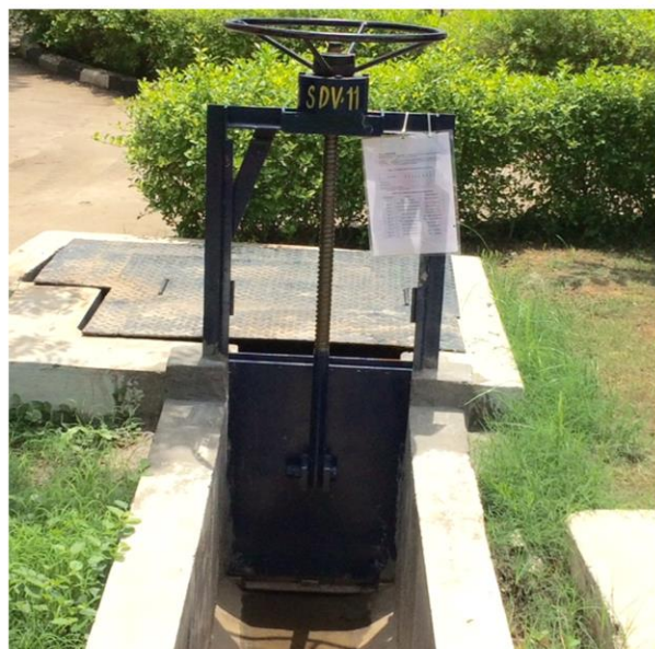
Sluice Valve at Strategic locations in storm drain
