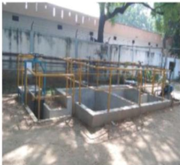
Guard Pond for Storm Drain
