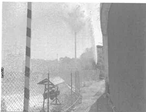
Fire Extinguishing by using Foam Monitor
